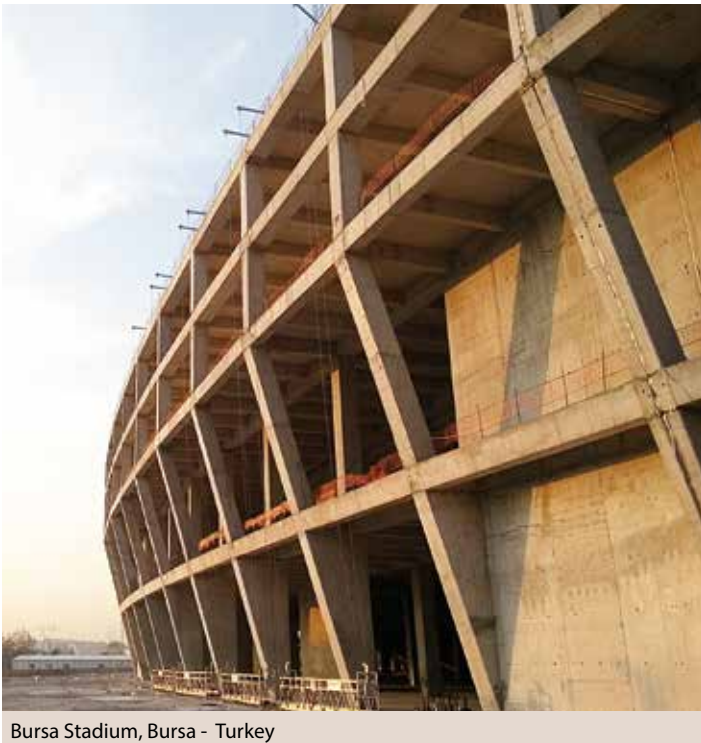
Bursa Stadium, Bursa - Turkey
