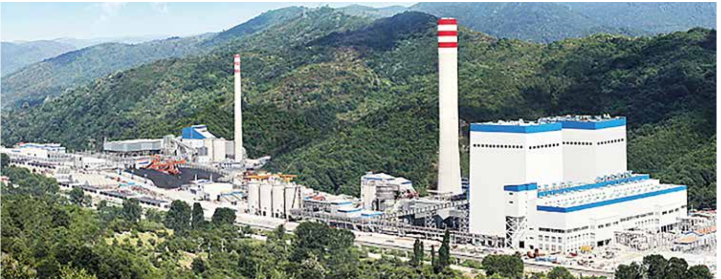
Eren Energy, Zonguldak - Turkey
