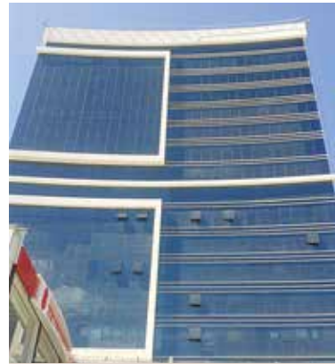
İstanbul Tower, İstanbul - Turkey
